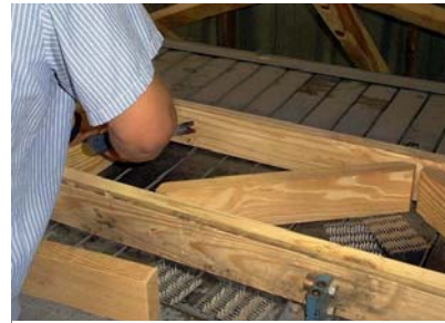
Set chords & webs into jigs
